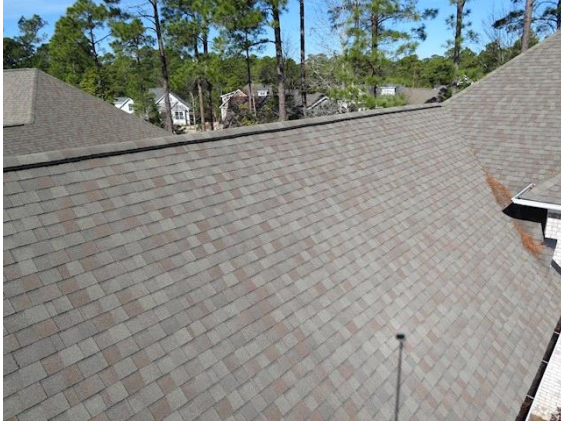
Roofing: Overall view of asphalt roof shingles
