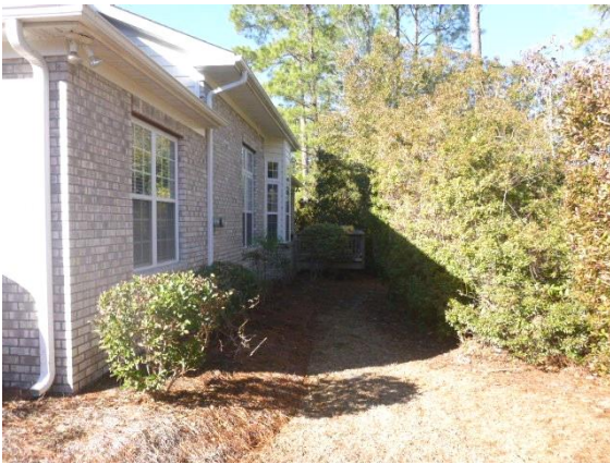
Grading / Drainage: View of rear property
