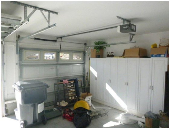
Overhead Garage Doors: Overall view of left garage door that did not operate
