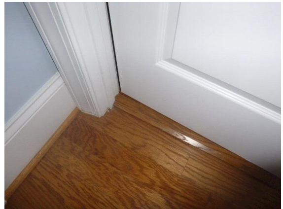
Bedroom #2 - Guest - Right Side - Front : View of entry door hitting threshold
