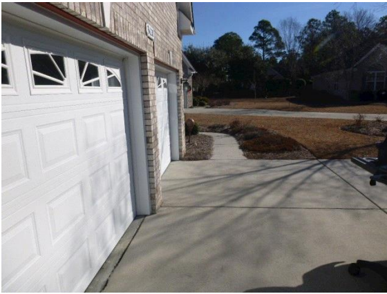
Grading / Drainage: View of front property
