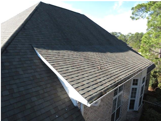
Roofing: Overall view of asphalt roof shingles
