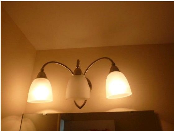
Bathroom #3 - Guest - 2nd Floor : View showing defective light in fixture located above the sink
