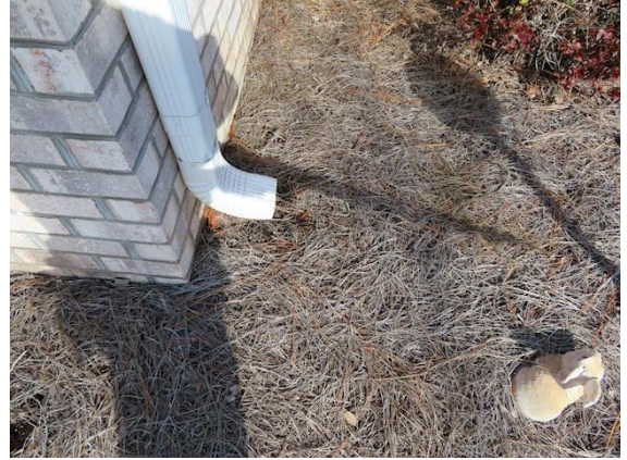
Gutters/Down Spouts: View showing one location of missing splash blocks/extension hoses at the end of downspouts
