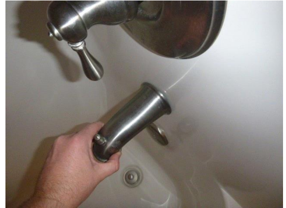
Bathroom #1 - Guest - Right Side : View of loose bath tub faucet
