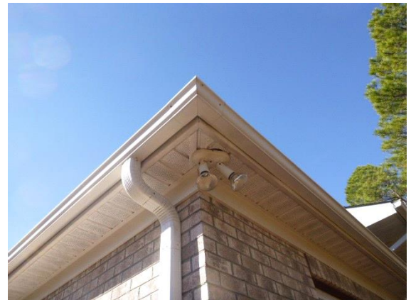
Exterior Surface: View of defective spotlight located at the right rear of house
