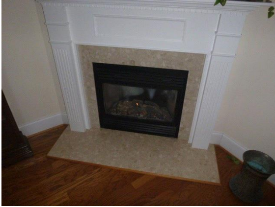
Fireplace/Stove: Overall view of fireplace
