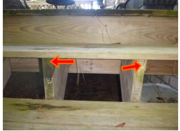
Walks / Steps: View of one location of cracked staircase stringers
