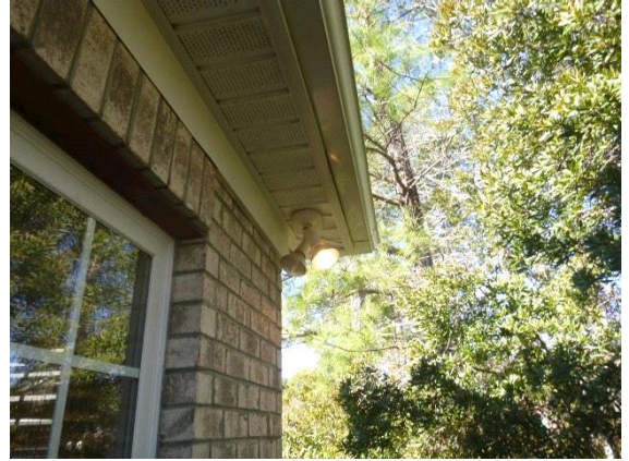
Exterior Surface: View of defective spotlight located at the left rear of house
