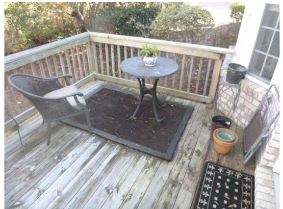
Decks / Balcony: Overall view of rear wood deck
