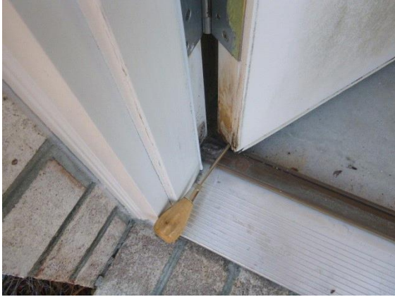
Exterior Doors: View of soft wood present at garage side entry door
