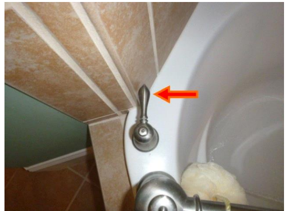
Bathroom #2 - Master: View of bathtub faucet handle hitting wall when operating
