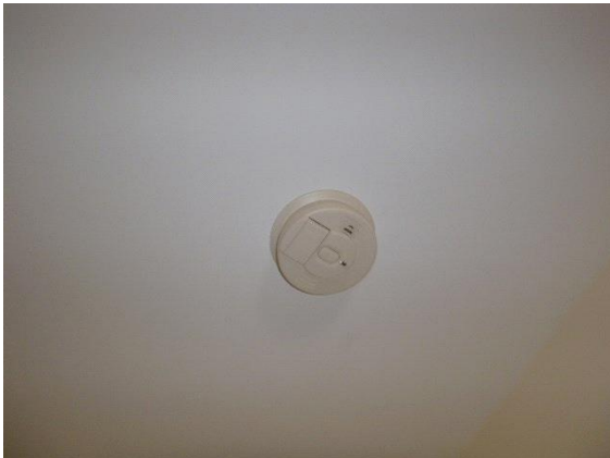
Electrical: All smoke detectors were checked and were operational at the time of the inspection
