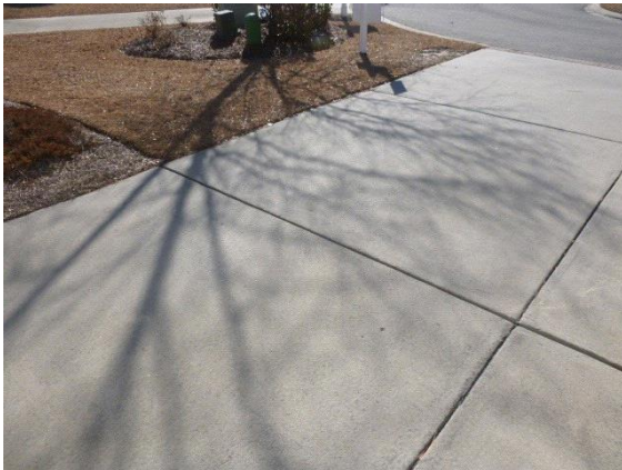
Driveway: Overall view of concrete driveway
