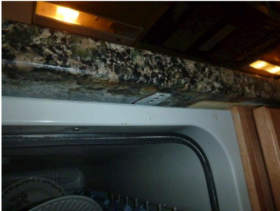
Kitchen: View showing the dishwasher tab not secured to the countertop
