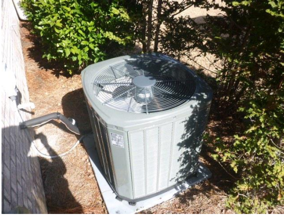
Heating: View of HVAC condenser located on the right side of house
