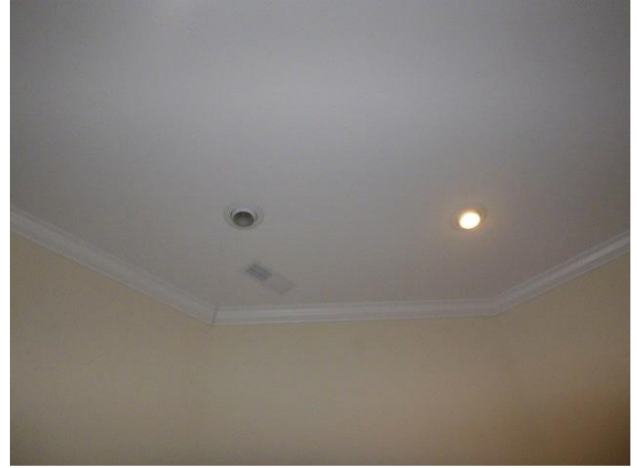
Living Room: View of defective light on living room ceiling
