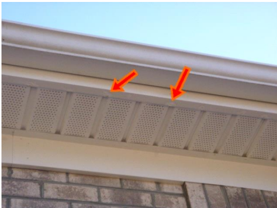
Exterior Surface: View of one location of peeling coated metal trim
