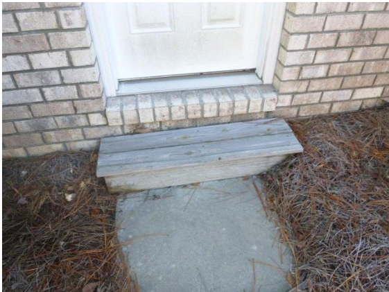
Walks / Steps: View of loose wood step at left side
