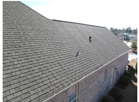
Roofing: Overall view of asphalt roof shingles
