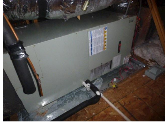
Heating: View of HVAC air handler located in the attic
