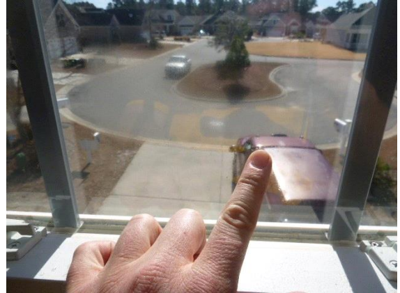
Finished Room Over Garage: View of fogged window
