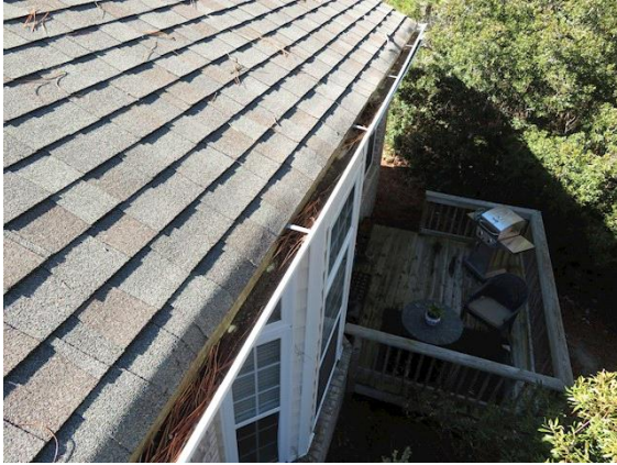
Gutters/Down Spouts: View of debris inside the roof gutters
