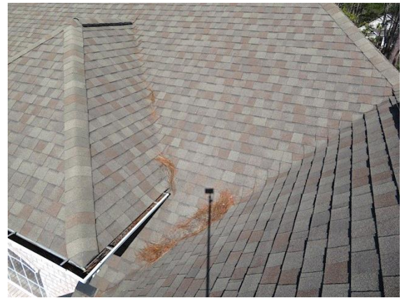
Flashing/Valleys: View of one location of debris in roof valleys
