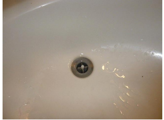
Bathroom #2 - Master: View of missing drain stopper in left side sink
