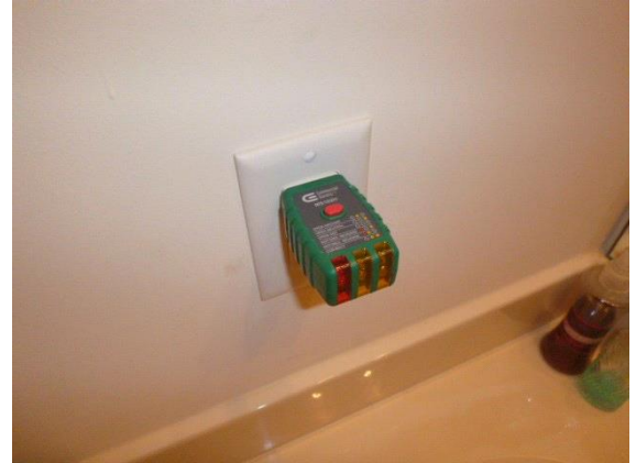
Bathroom #3 - Guest - 2nd Floor : View of no power present at GFCI receptacle in bathroom
