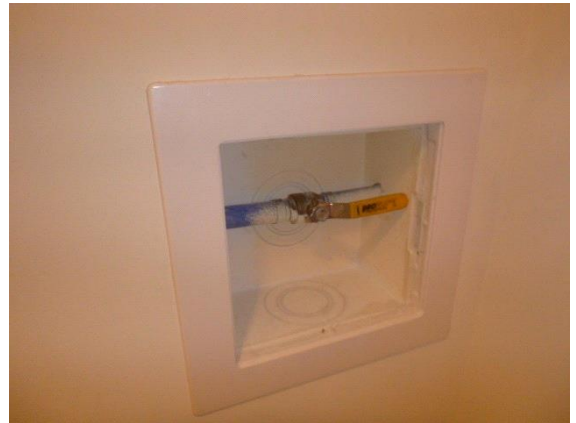
Plumbing: View of main water shut off valve located in the laundry room
