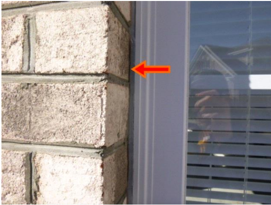
Windows: View of one location of separated caulking at windows
