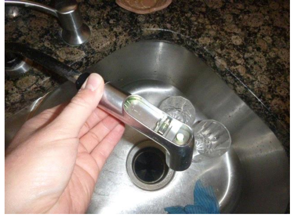
Kitchen: View of hand sprayer missing control button
