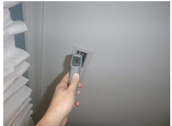
Heating: View of supply air temperature using a digital thermometer in the heating mode
