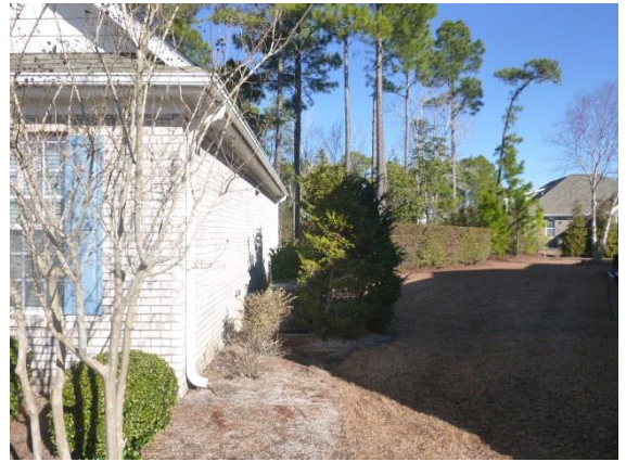
Grading / Drainage: View of right side property
