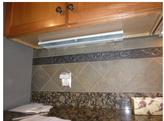
Kitchen: View of one location of defective kitchen light fixture
