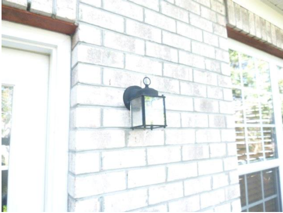
Exterior Surface: View of defective light fixture located next to rear entry door
