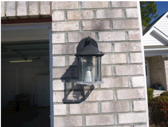
Exterior Surface: View of defective light fixture located next to garage roll up door
