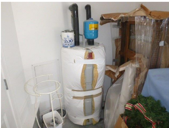
Water Heater: View of insulation installed on water heater
