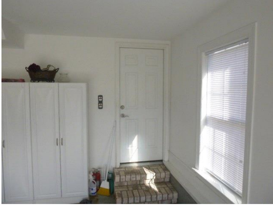
Garage Pedestrian Door into House: Overall view of garage pedestrian door
