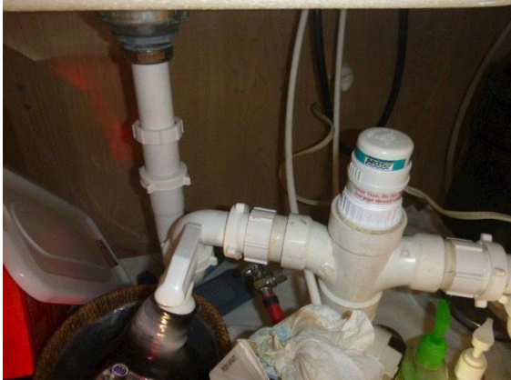
Plumbing: View of plumbing pipes below sinks
