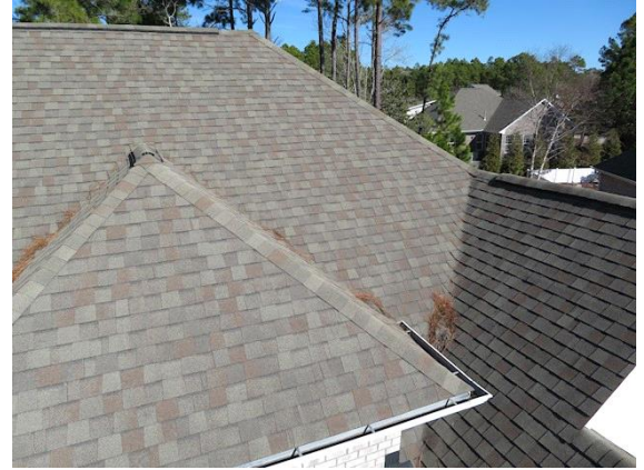
Roofing: Overall view of asphalt roof shingles
