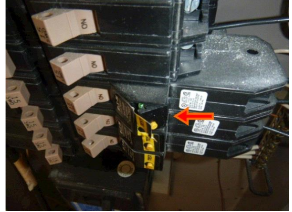
Electrical: View of damaged Arc Fault breaker
