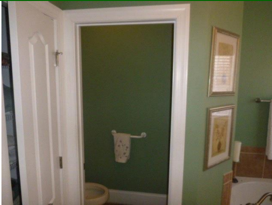
Bathroom #2 - Master: View of missing toilet closet door
