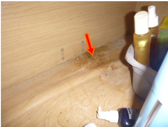
Bathroom #2 - Master: View of water damage to particle board located under the bathroom sink
