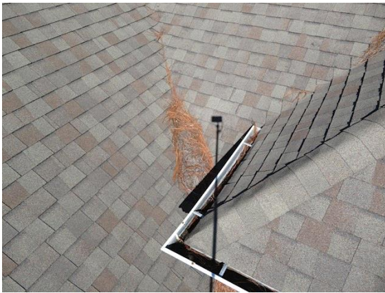
Flashing/Valleys: View of one location of debris in roof valleys
