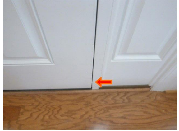
Exterior Doors: View showing daylight between front entry door and door jamb
