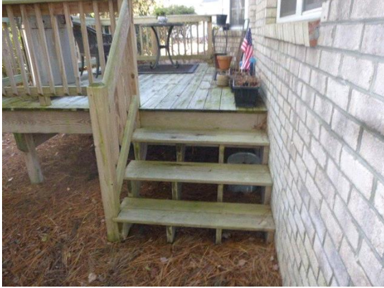
Walks / Steps: Overall view of rear wood steps
