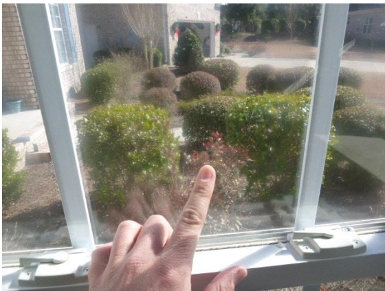
Garage/Carport: View of fogged window located in the garage
