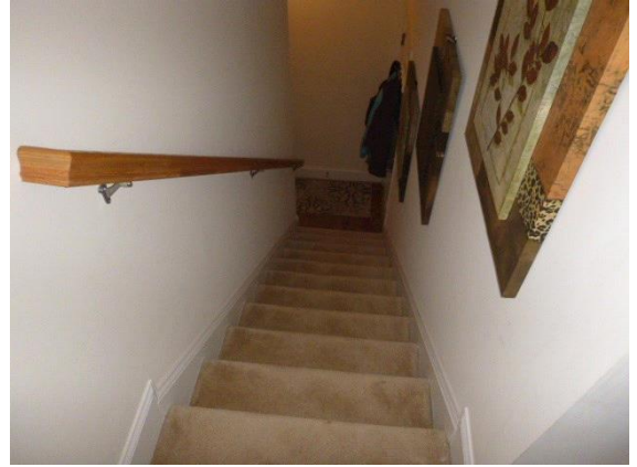
Stairs / Railings: Overall view of interior stairs and railings
