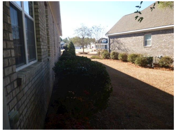
Grading / Drainage: View of left side property
