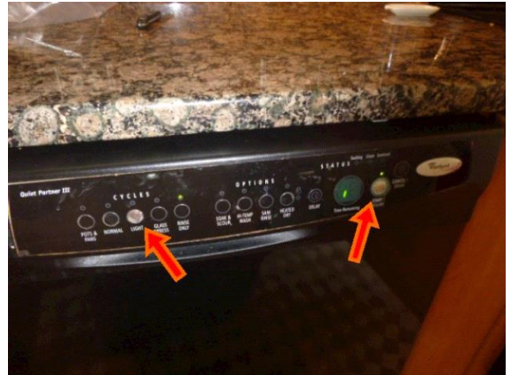
Kitchen: View of damaged dishwasher control buttons
