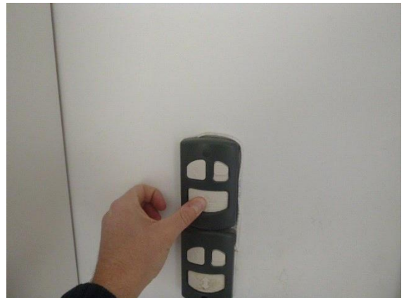
Overhead Garage Doors: View testing left side garage door opener
